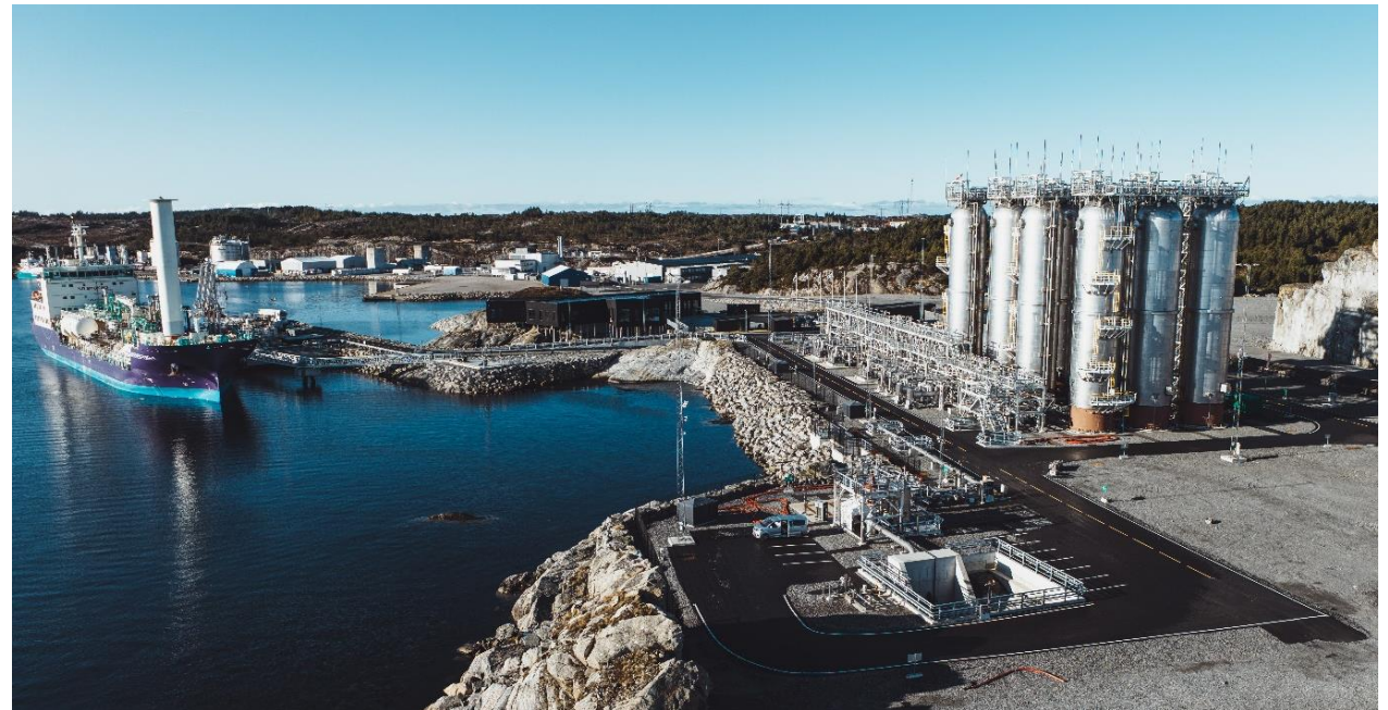
Example of a Northern Lights vessel at an unloading terminal in Norway ( https://norlights.com/about-the-longship-project/ )
